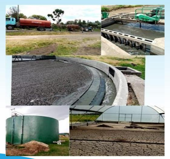
From the MDU the fecal sludge is transferred into a primary collection point and subsequently towered to the treatment plant where it is emptied into the sewer treatment plant for further treatment and processing into bio-fuels products.
