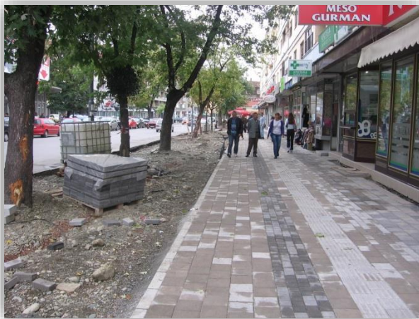
Reconstruction of sidewalks with use of tactile tiles
