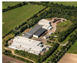
Biogas- und Kompostwerk Bützberg: Dry fermentation and composting plant with triple – strategy (gas prod., storage-grid, compost)
